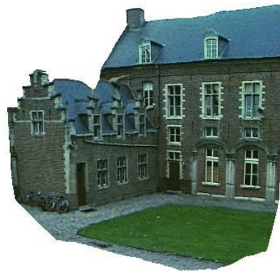
Figure 14.8. A synthetic texture-mapped image of a castle constructed via projective motion analysis followed by metric upgrade. The principal point is assumed to be known. Reprinted from [?], Figure 6.13.
